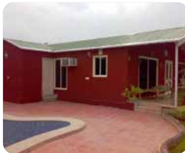
PREFAB FARM HOUSE
